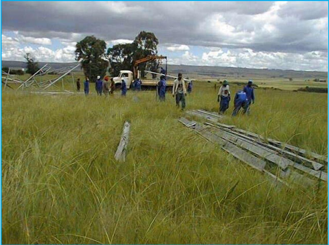
Figure 3-9: On-site erection of towers
