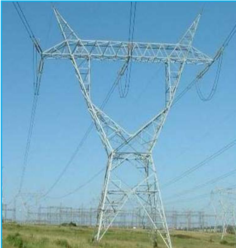
**Figure 3-2: Self-supporting Pylon**
