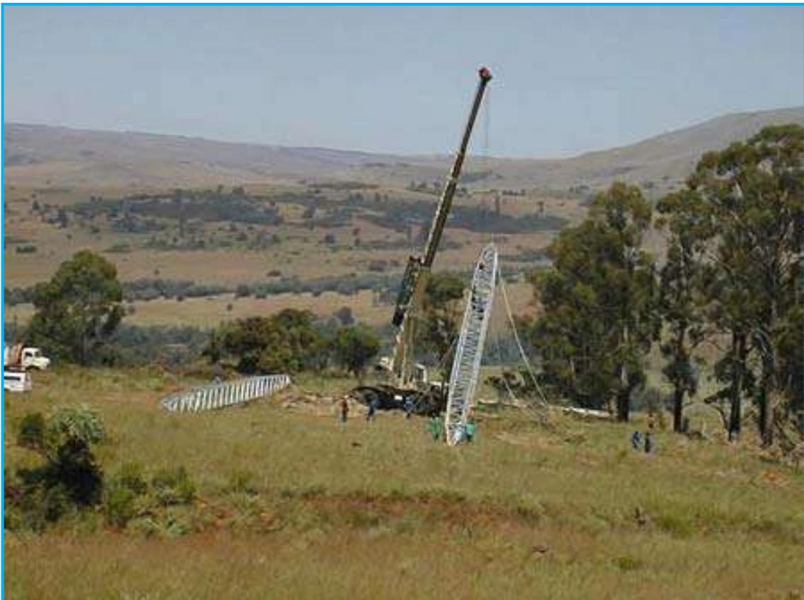
Figure 3-10: Erection of towers by crane
